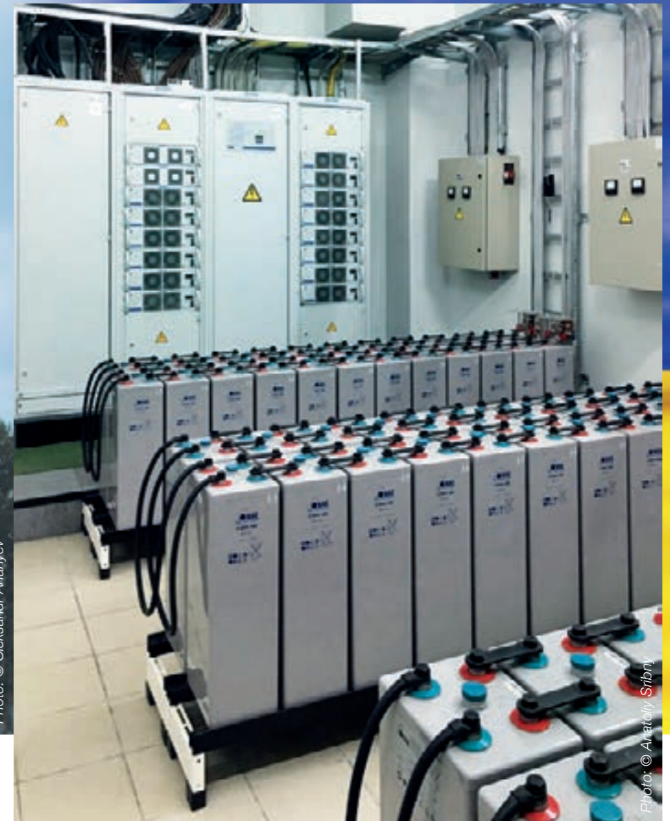
The rear cabinet series has a 48 V / 216 kW telecommunications system with TEBECHOP 13500 modules consisting of module cabinets, mains supply fields as well as battery and load output fields, including a monitoring system. The front contains the battery system, along with battery connection boxes.
