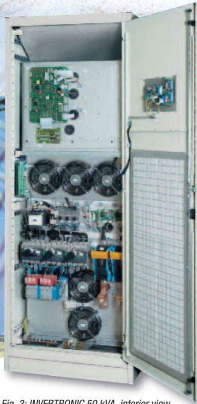
Fig. 3: INVERTRONIC 50 kVA, interior view
